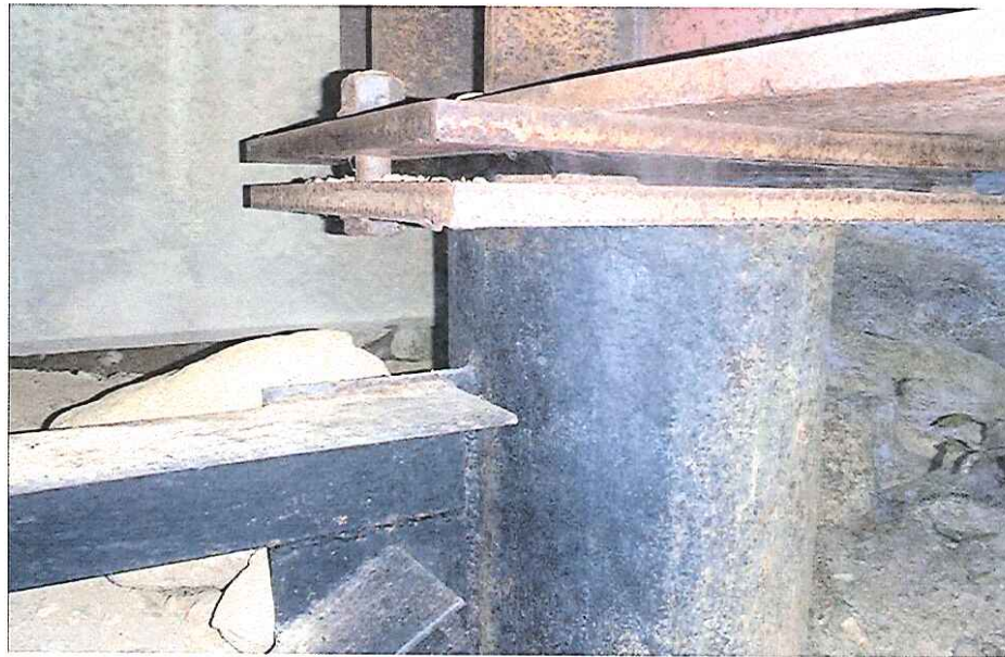
CK2285 Right Abutment bearing
