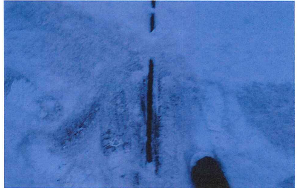
CK2285 Deck joints
