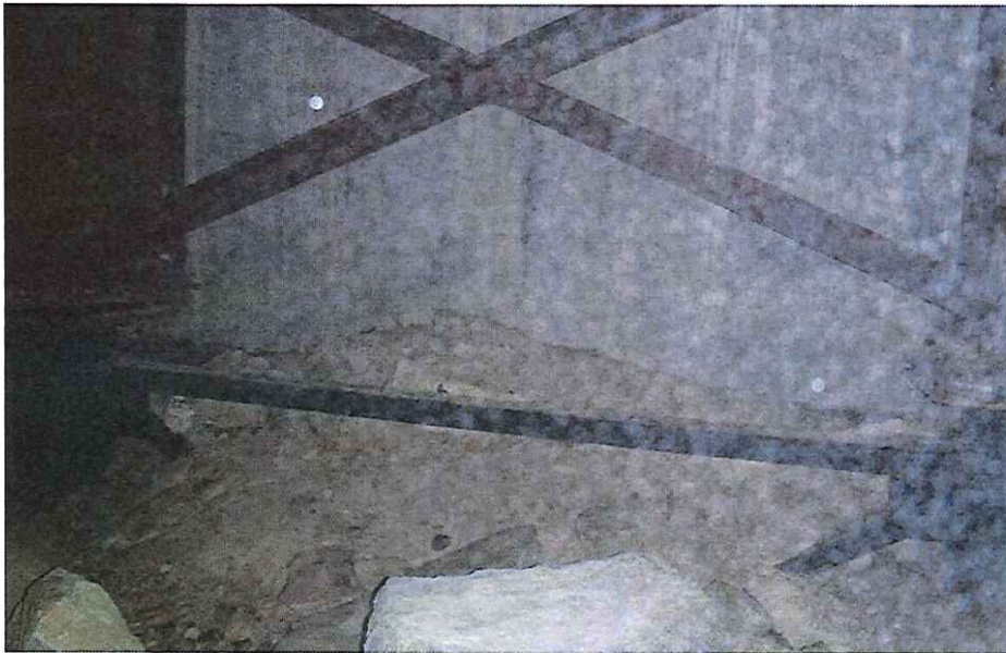
CK2285 Right Abutment
